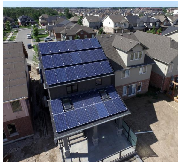
Image 2: Back elevation of Reid’s Heritage Homes’ Net Zero Energy Home showing the solar photovoltaic
