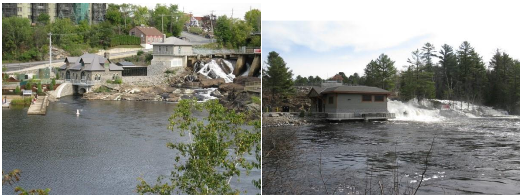
Bracebridge Falls Generating Station (left) and Wilson's Falls Generating Station (right).
